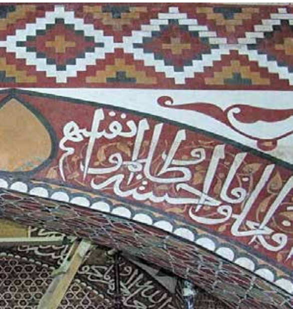
Minor dome, hatching, retouching and simplification of a floral pattern (above)
