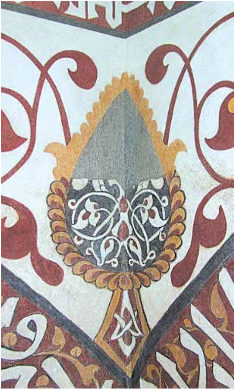
Minor dome, hatching, retouching and simplification of a floral pattern (above)
