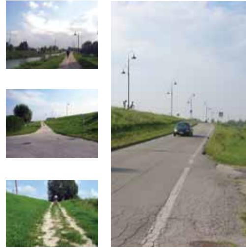
roads and dike paths are built on top of levees; safety and access are both problematic
